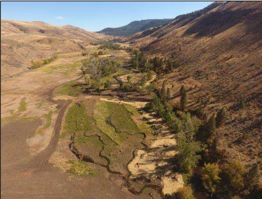
CONSTRUCTION OF LARGE WOOD STRUCTURE AT LOWER PROJECT AREA.
