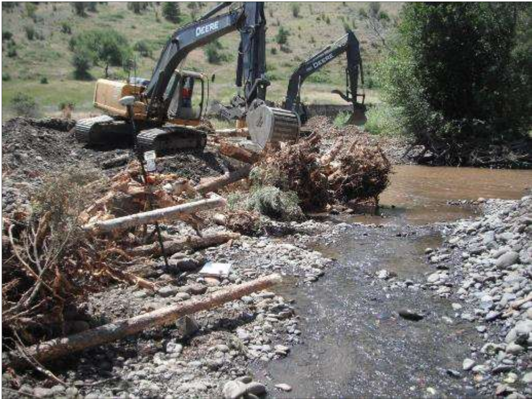
CONSTRUCTION OF LARGE WOOD STRUCTURE AT UPPER PROJECT AREA.
