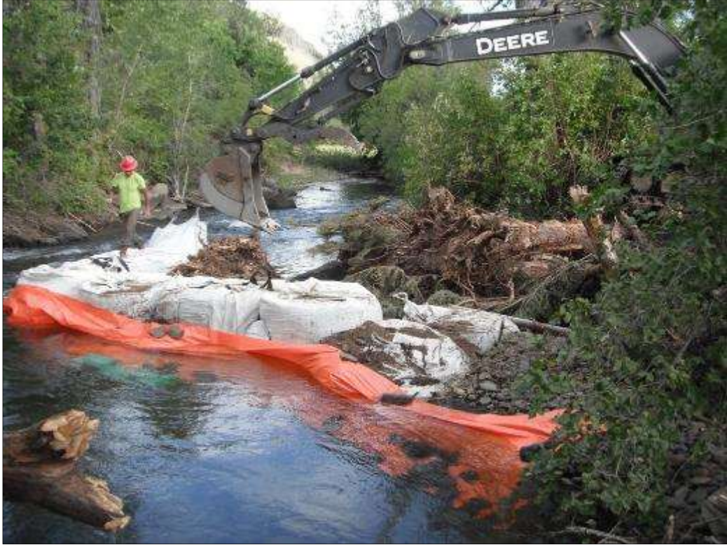
CONSTRUCTION OF LARGE WOOD STRUCTURE AT UPPER PROJECT AREA.
