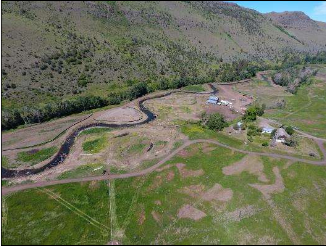
TWO PHOTOGRAPHS OF SOUTHERN CROSS CONSTRUCTION AT THE UPPER AND MID PROJECT AREAS JUNE 2016 AND SEPTEMBER 2016.
